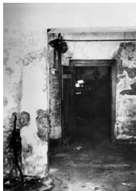
Figure 18.2 A “bunker” in the cellar of the assembly camp
