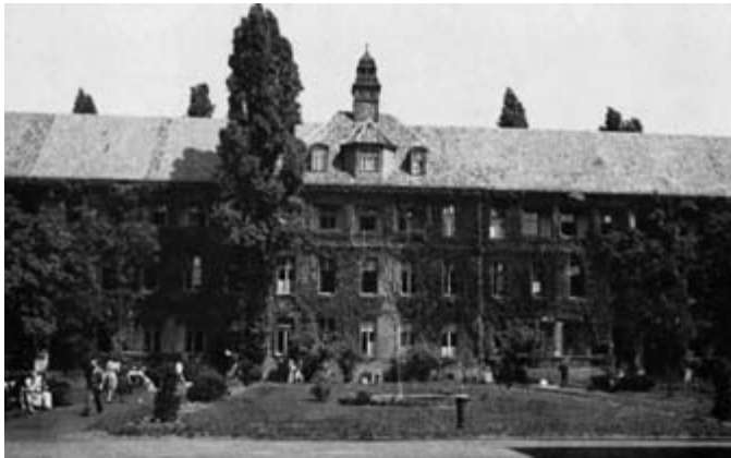
Figure 18.4 The main building of the Jewish hospital in the 1930s
