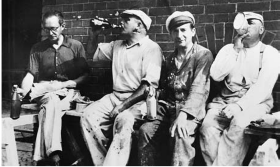
Figure 8.2 Jewish forced laborers from the Hensel family on a lunch break from building the air-raid shelter for the Community school on Richard-Wagner-Strasse
